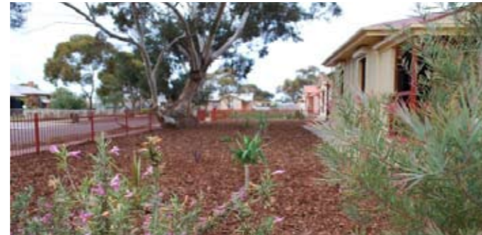
Renovated Nunuyara Health Clinic
